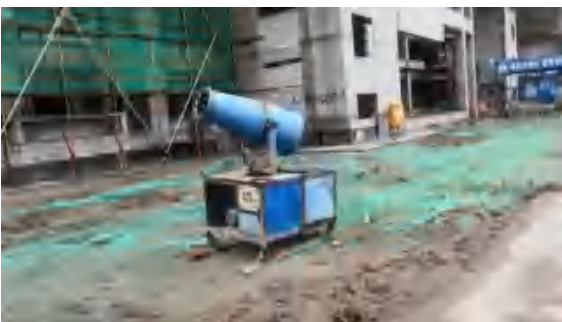
裸露场地密目网苫盖 (2020.05)
