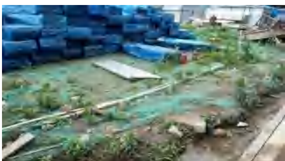
施工场地密目网苫盖 (2020.05)
